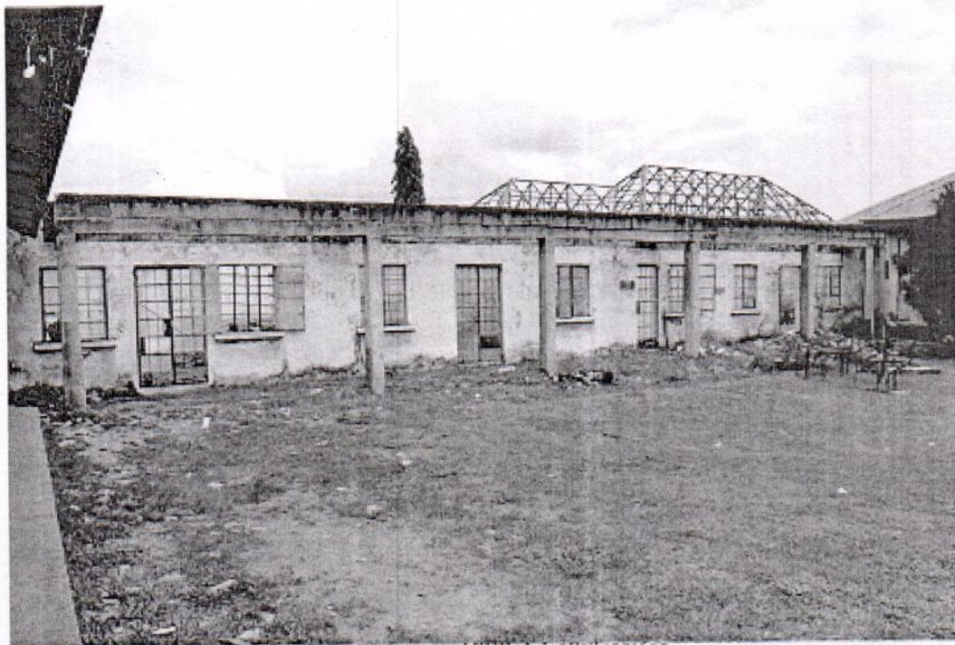
RENOVATION OF CEFTER BLOCK
